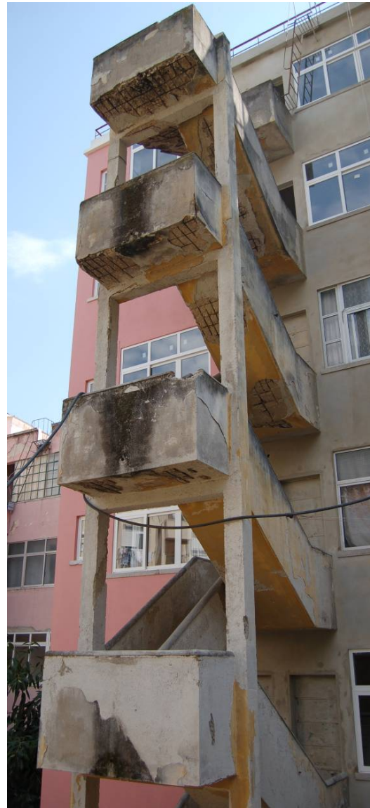
Figure 2: Front/right side view of the stairs
