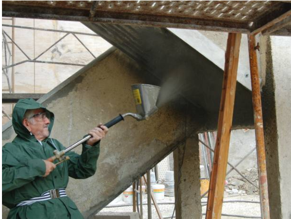
Figure 5: Spraying PCM of SB
