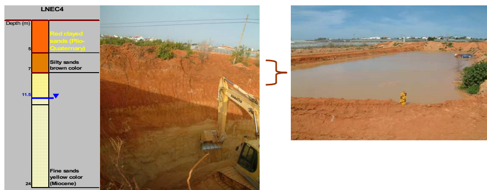
Figure 1 –Vertical profile of lithological materials in Areal Gordo (at right) and LNEC4 well lithological column and, infiltration basin in the first layer (at left)
