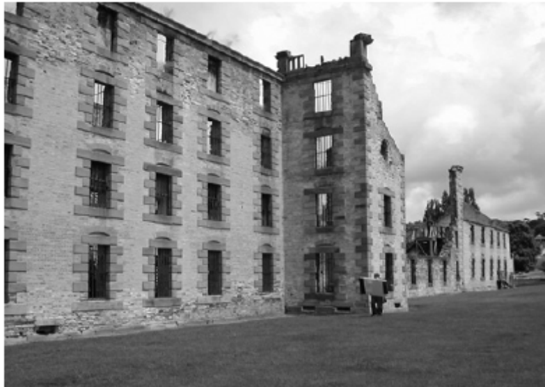
Figure 4: The penitentiary building of the Port Arthur Historic Site. © Marta de la Torre, GCI. The management of the site for the past decade is regarded as a successful example of the application of the Burra Charter Process, which submits decisions to the preservation of the site significance while fostering negotiation among stakeholders and providing enough latitude for the consideration of economic viability concerns.
