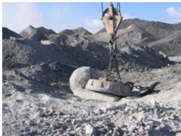
FIG. 4—Breaking up equipment of steel slag (Roque et al., 2007).
