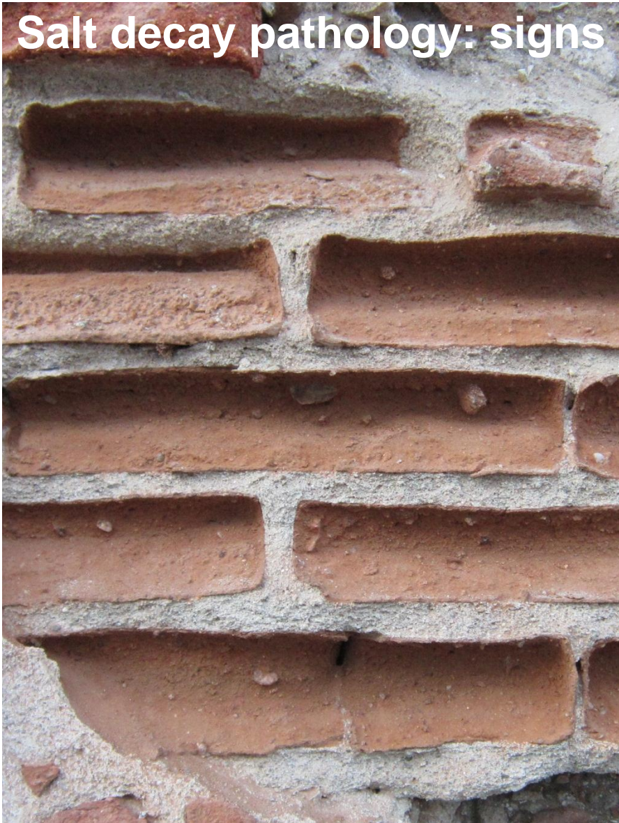
Powdering of ceramic bricks
