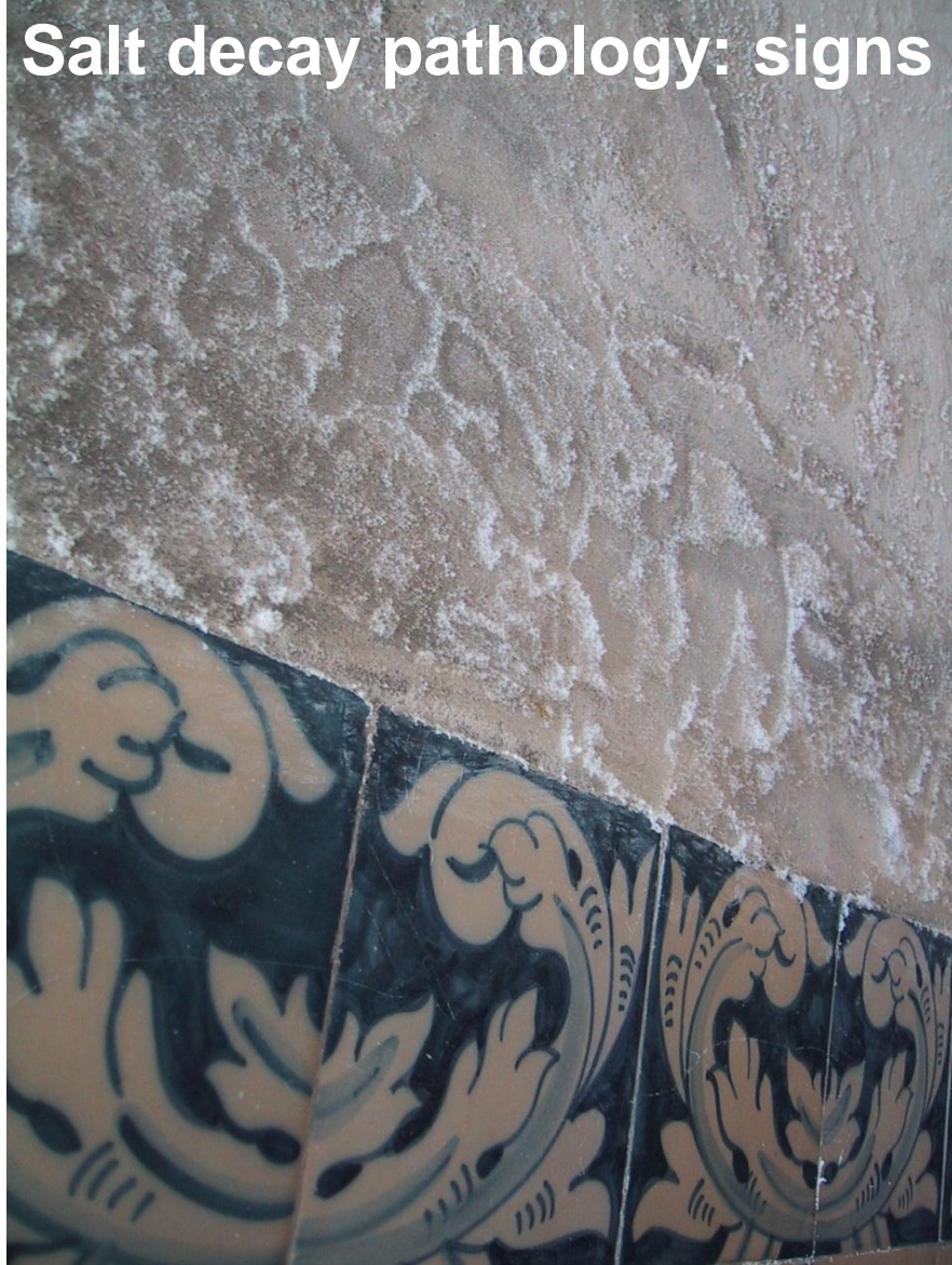
Efflorescence
