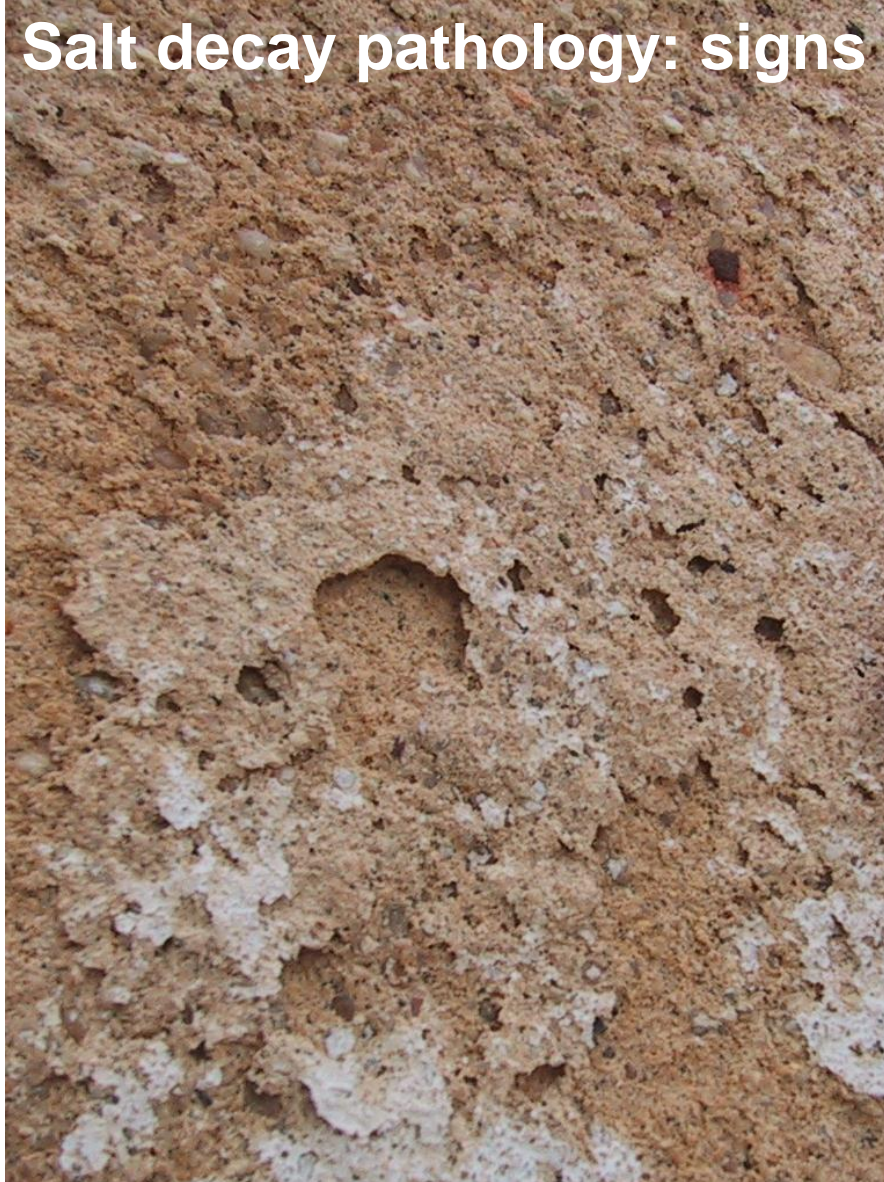
Scaling of the lime-wash/ lime render system
