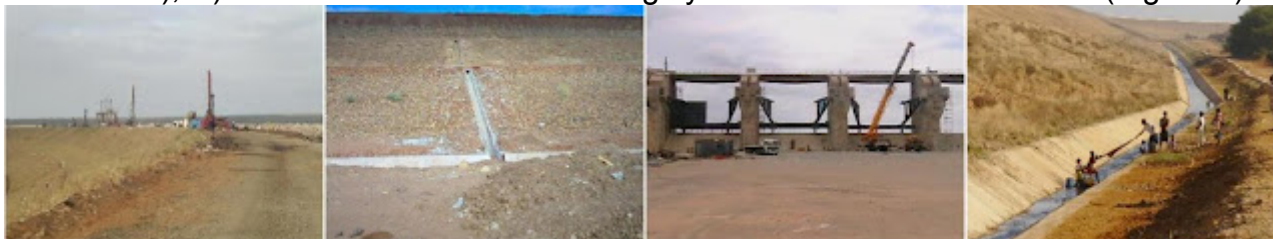
Figure 4 - Rehabilitation works: injections, stabilizing berm, gates and relief wells and ditch
