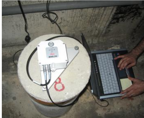
Figure 15 – Inclinometer setting up: computer
