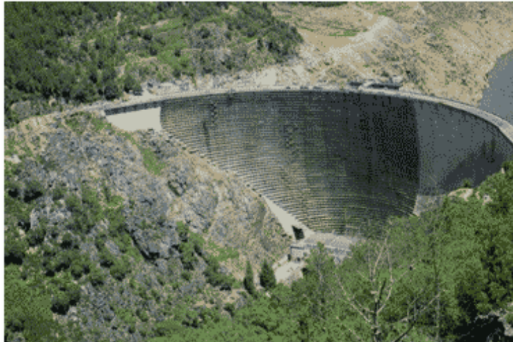
Figure 13 – Repair works in Cabril dam
