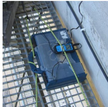
Figure 17 – Digital thermo-hydro-barometer on the walkway
