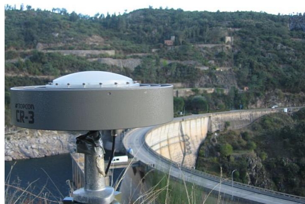
Figure 2 – GNSS antenna (reference point) during the continuous monitoring test
