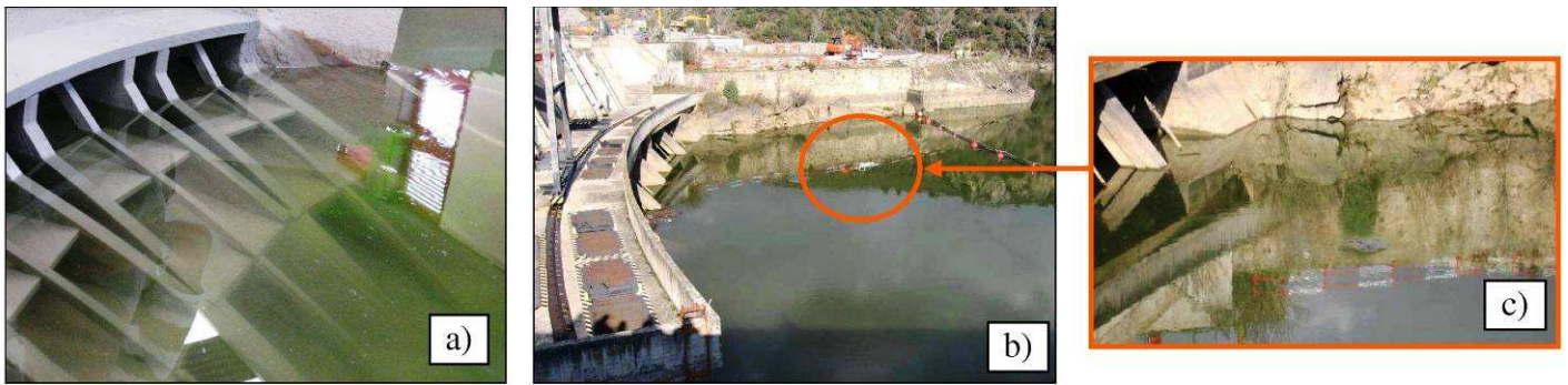
Fig. 5 – Vortice near the water intake of the old power circuit. a) physical model of Bemposta dam; b) and c) prototype
