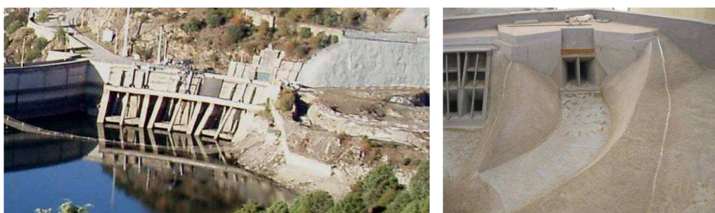
Fig. 3 - Bemposta dam. Approach channels and water intakes of the two power stations, old one at left (prototype) and new one for the reinforcement at right (physical model).
