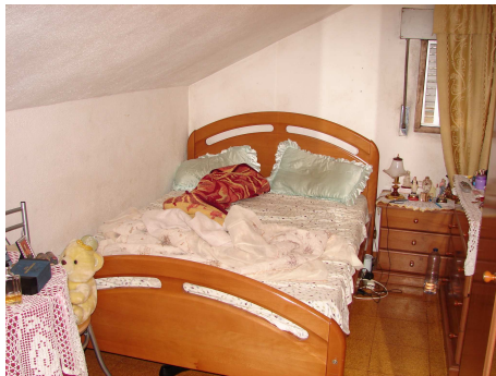
Figure 7. Bedroom with low ceiling height.
