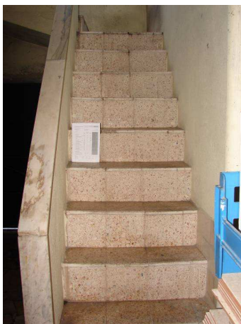
Figure 4. Stairs with high rise steps.
