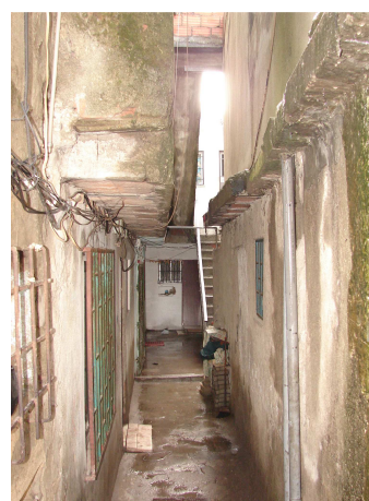
Figure 3. Windows opened to an alley with about 1 meter width.
