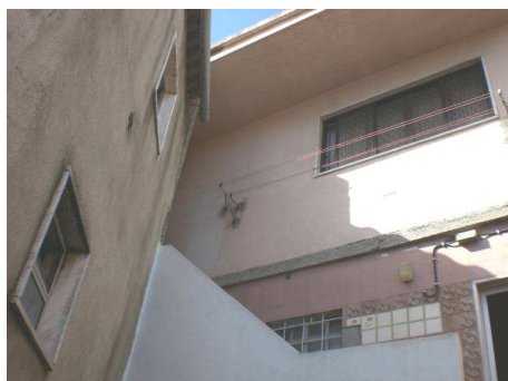
Figure 2. Small distance between windows of neighbouring buildings.
