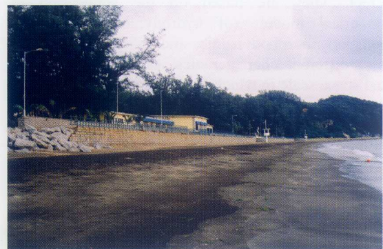
Figure 2. Vertical seawall at Hac-Sá backshore.
