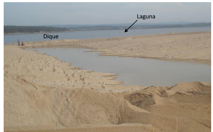
Figura 3. Dique (na margem interna da barreira) e vala escavada durante a operação de abertura artificial da embocadura. Figure 3. Sandy dike on the internal margin of the barrier, and excavated trench during the opening works of the artificial inlet.
