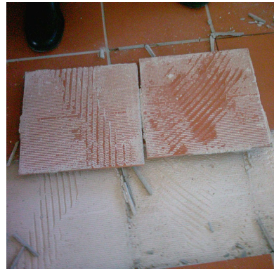
Figure 2: Back of detached tiles
