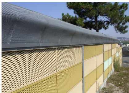
Figure 3 – Cylindrical diffracting edge developed by Complage
