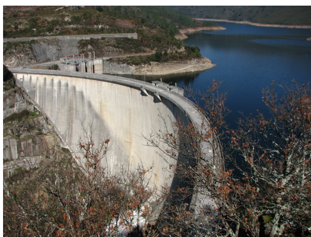
Figure 4: Alto Lindoso dam
