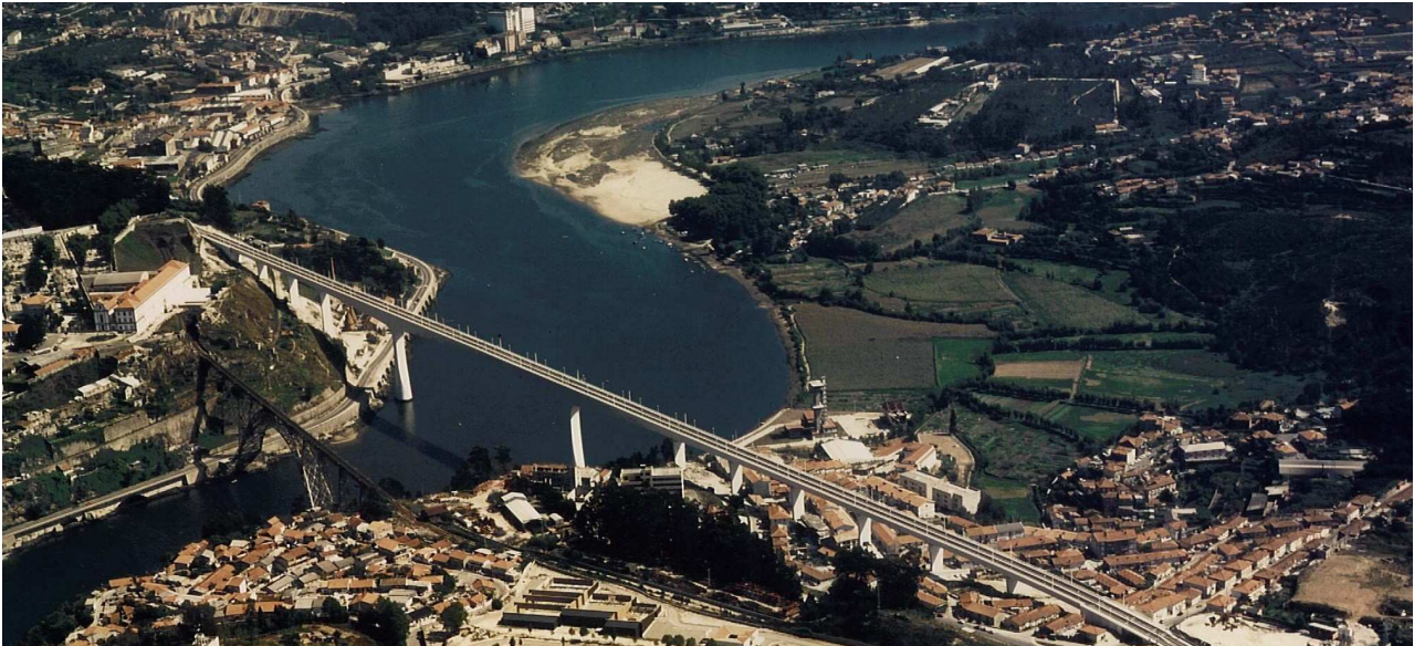
Fig. 2: General view of São João Bridge
