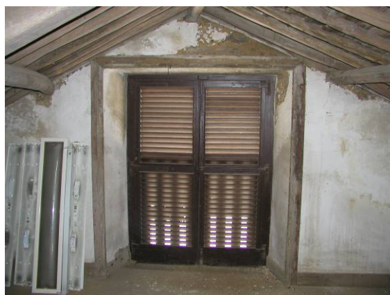
Figure 2: Example of a possible point of entry of C. brevis alates
