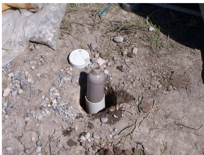
Fig. 8 - Piezometer installed for ECOMANAGE project
