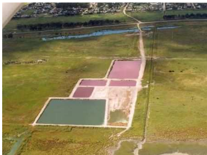
Fig. 41 - Siracusa slaughterhouse's water treatment plant
