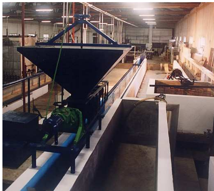
Figure 3.3 Coarse sediment feeder
