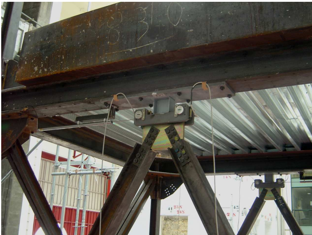
Figure I.2: Detail on the Dorka device (South).
