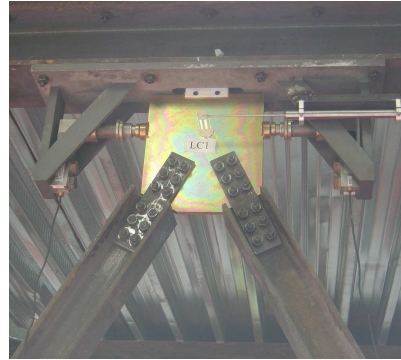
Figure 17: View of Jarret's viscous fluid damper.
