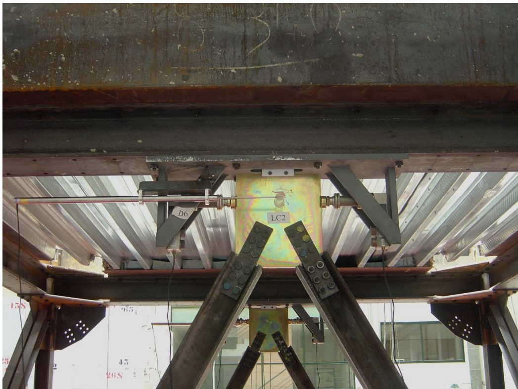
Figure I.12: Detail on the Jarrett device (South).
