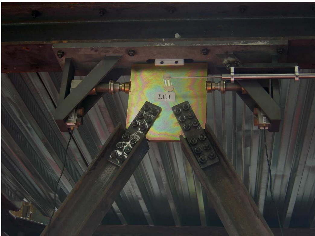
Figure I.10: Detail on the Jarrett device (North).
