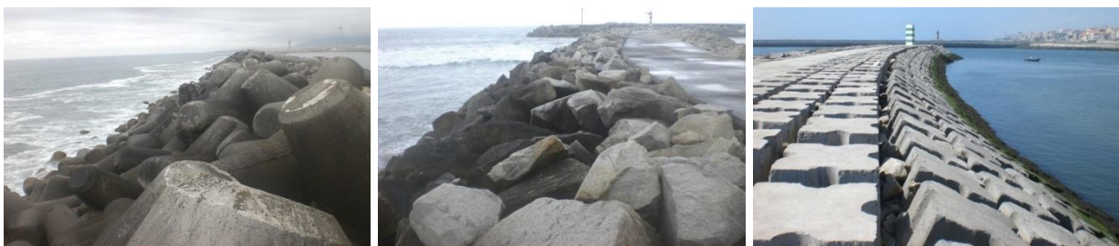
Fig. 1. Breakwater armor layers composed of a) rock units (Vila Praia de Âncora); b) and c) concrete units (Viana do Castelo, Foz do Douro)
