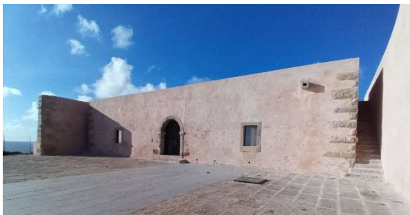
Fig. 4. Paimogo Fort after the intervention work, in 2025.
