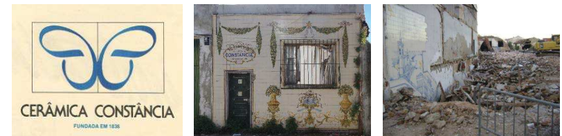
Figure 1. Constância Ceramic factory. Left: factory logo; Middle: entrance to the factory facilities/shop before demolition; Right: after the demolition (Image by Pinto Soares)
