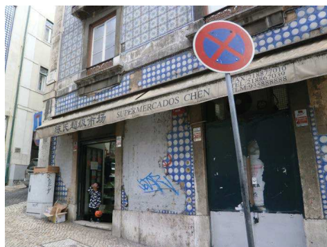
Figure 1. Lack of maintenance, loss of tiles and unappropriated interventions.
