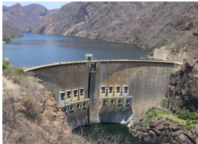
Figure 1.1: Downstream view of Cahora Bassa dam
