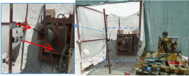
Figure 1. General view of a ground nail load test layout.
