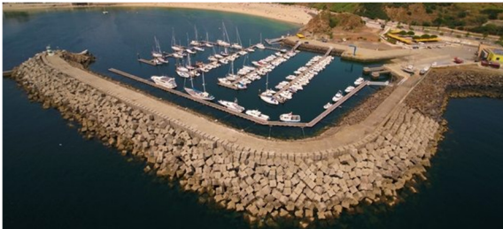
Figure 2: Breakwater of the leisure port of Sines.
