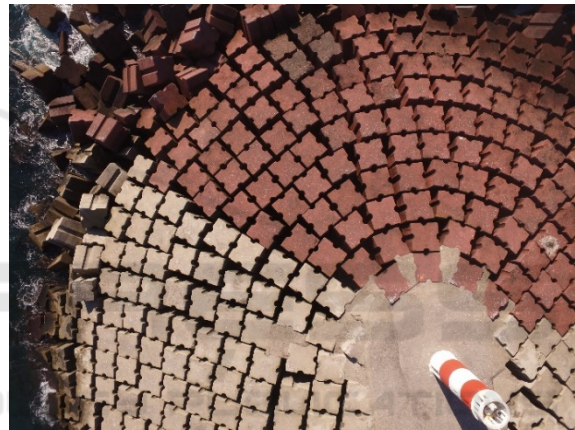
Figure 5: The head of Sines west breakwater.
