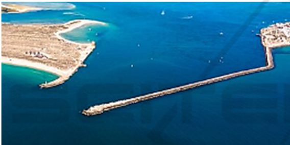
Figure 3: Breakwaters of Faro-Olhão inlet.
