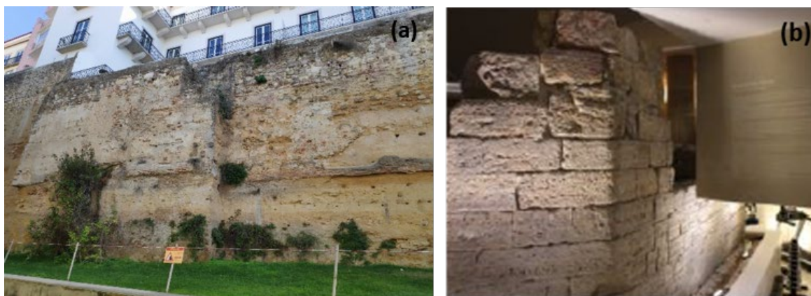
Figure 4. Case studies in Wall Western fluvial section: Terraços de Bragança Complex (a) and Corpo Santo Hotel (b).
