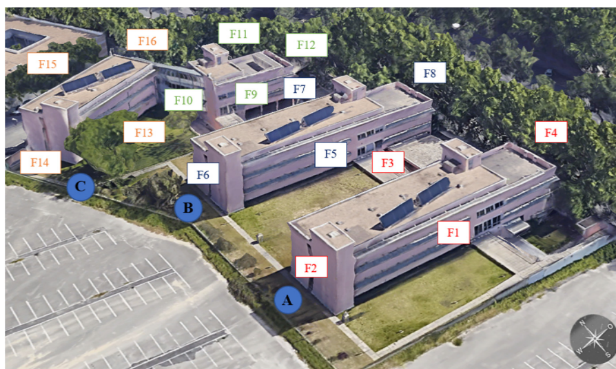
Figure 2. Representation of the inspected building complex identifying the 16 façades (credit: Google Earth).
