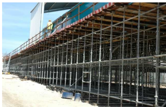
Fig. 1: Example of bridge falsework Cuplok® systems
