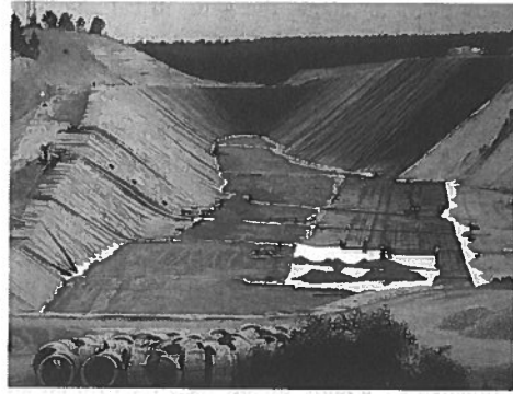
Fig. 3. General view of the landfill.
