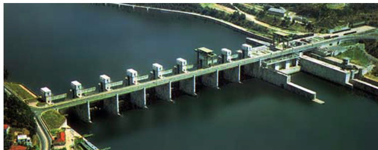
Figure 2. Crestuma-Lever dam aerial view.
