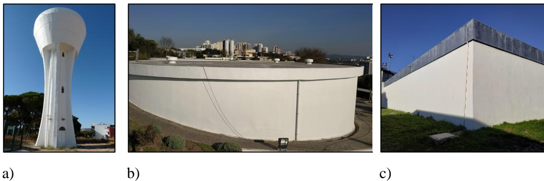
Figure 3.2 – Examples of tank typologies: a) frustoconical water tower; b) circular cross-section half-buried tank; c) rectangular cross-section tank.
