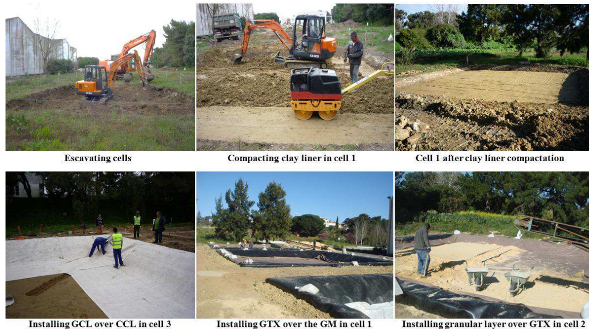
Figure 2. Pilot plant construction
