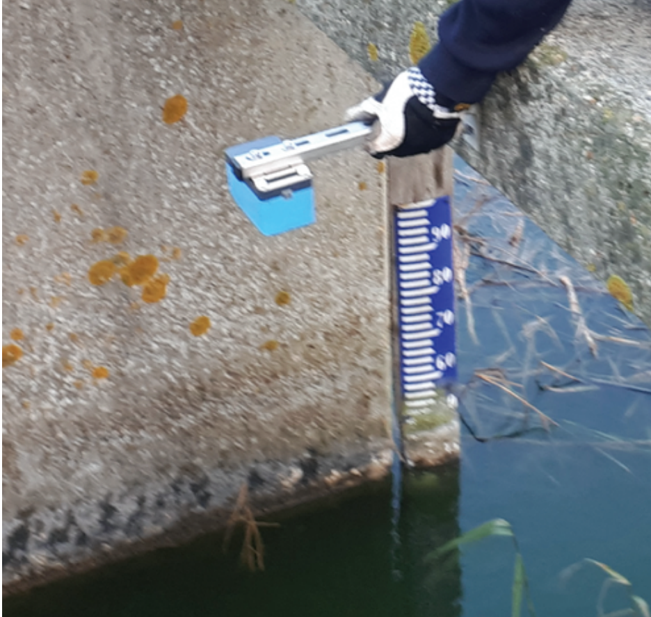
Figure 3. Staal water surface level sensor.
