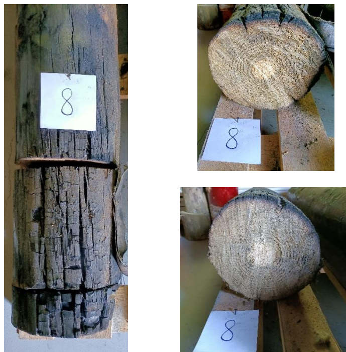
Figure 3.13 – Bottom end of pole 8 – Solution fire retardant fabric & treated pole (left – bottom end of the pole; right up – Cross-section at 10cm of the end; right bottom – Cross-section at 30 cm of the end)
