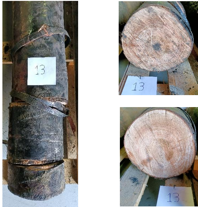
Figure 3.14 – Bottom end of pole 13 – Solution fire retardant fabric (left – bottom end of the pole; right up – Cross-section at 10cm of the end; right bottom – Cross-section at 30 cm of the end)
