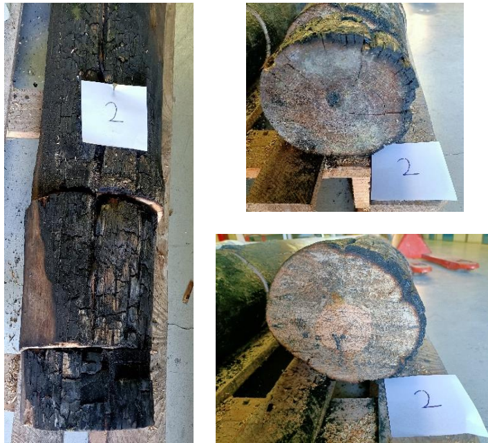
Figure 3.6 – Bottom end of pole 2 – unprotected & untreated pole (left – bottom end of the pole; right up – Cross-section at 10cm of the end; right bottom – Cross-section at 30 cm of the end)
