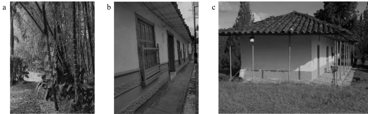
Fig. 1. (a) Guadua; (b) Wattle and daub house; (c) Rammed earth house
