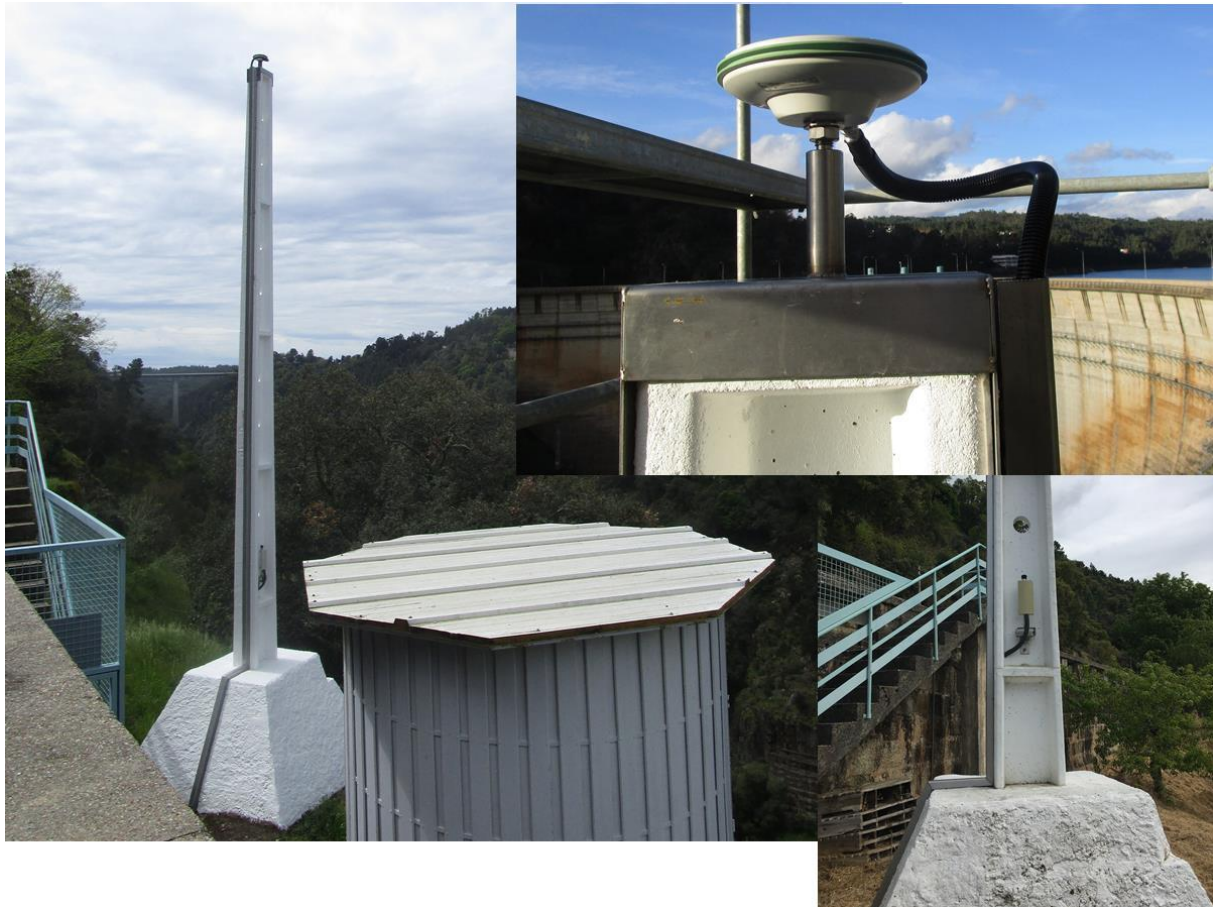
Fig. 3 – The GNSS reference station monument (on left, a general view, on top right, the top of the pillar with antenna GNSS, on bottom right, the pillar base)
