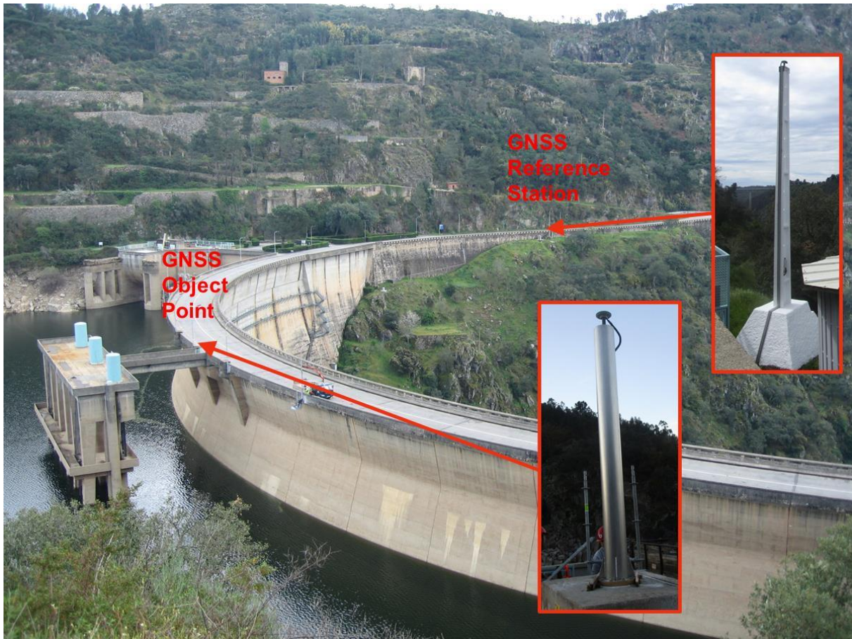
Fig. 2 – Location of GNSS stations in the Cabril dam: Reference Station, left bank, and Object Point, crest of the dam
