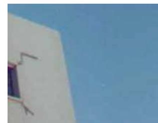
Figure 8. Cracking in window corners, in last floor, due to effect of temperature variations
