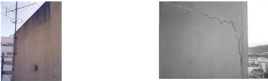
Figure 1. Example of cracking situations associated with the effects of temperature variations
