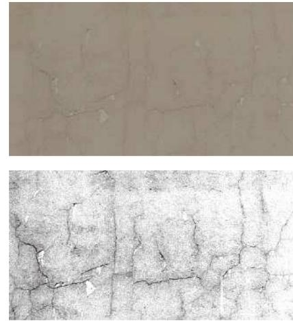
Figure 5 - Detail of an orthomosaics of a facade (top) and the enhancement, by image processing techniques, of the cracks on the surface (bottom)
