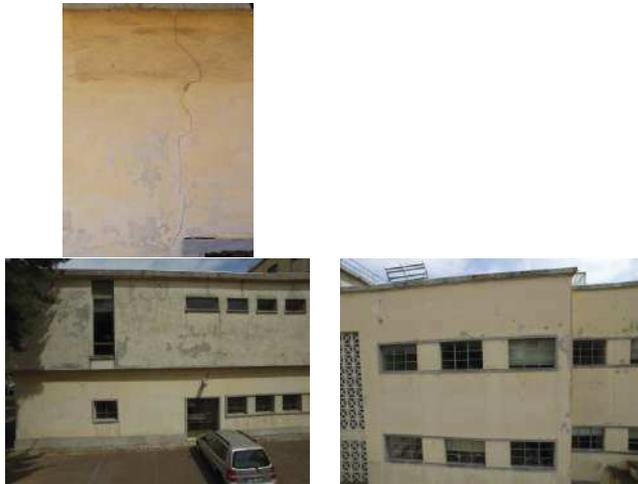
Figure 4 - Photos taken by the drone of building facades with signs of cracking that can probably associated, in part, to temperature variations [6]
