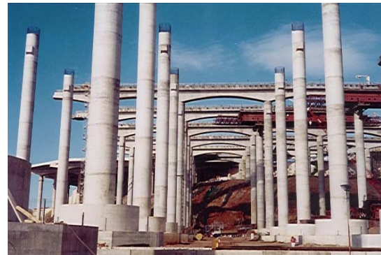
Figure 2. The runway extension in construction
