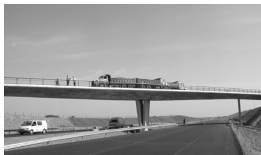
Figure 8. The truck loads on the central pier
