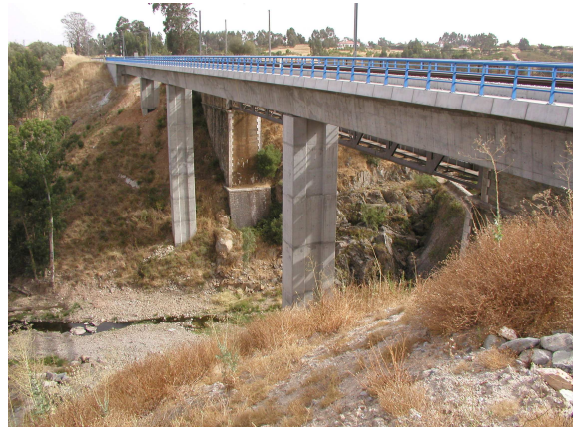
Figure 4. General view of Espinhaço de Cão Bridge
