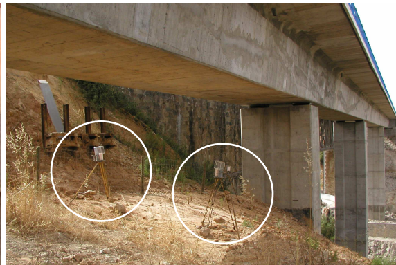
Figure 7. Deflectographs at Espinhaço de Cão Bridge
