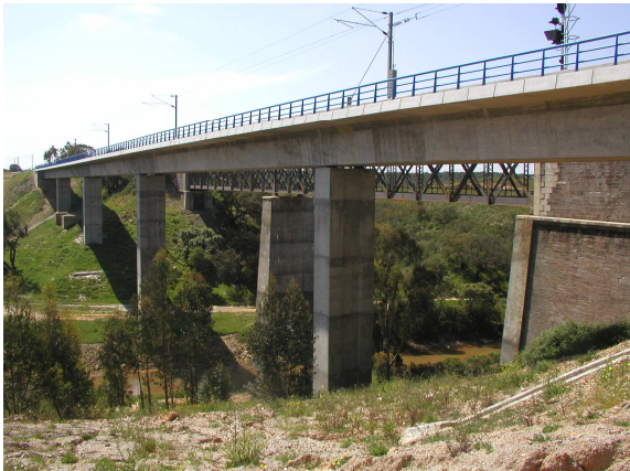
Figure 3. General view of Corona Bridge
