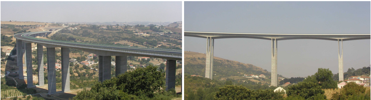
Fig. 2 General views of Loureiro Viaduct
