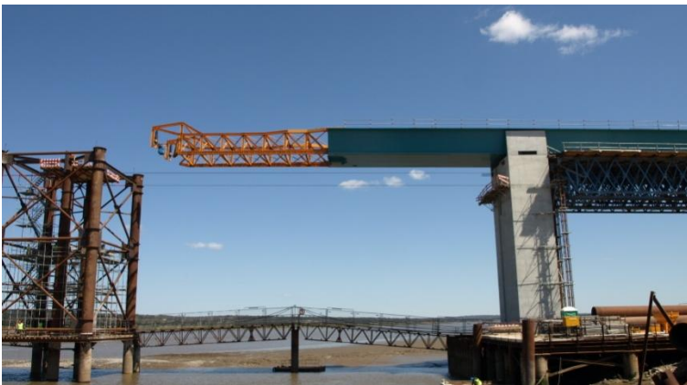
Fig. 2: Deck incremental launching
