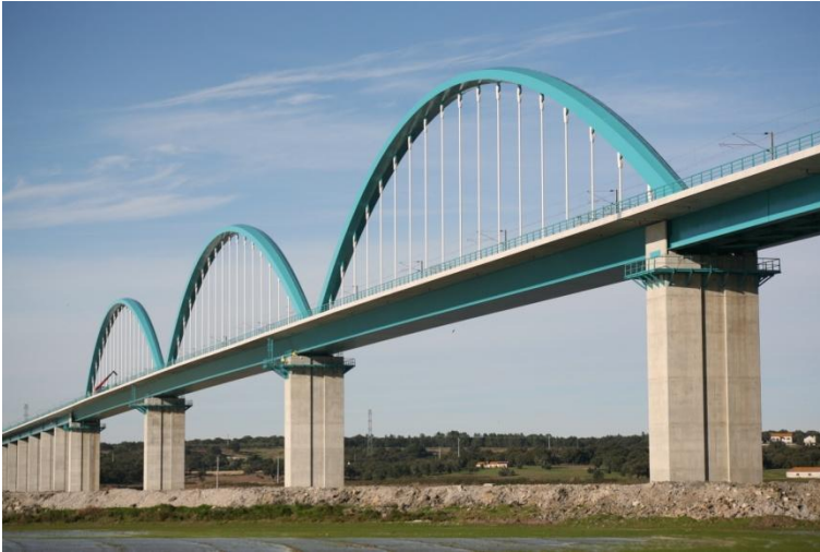
Fig. 1: General view of the bridge over River Sado
