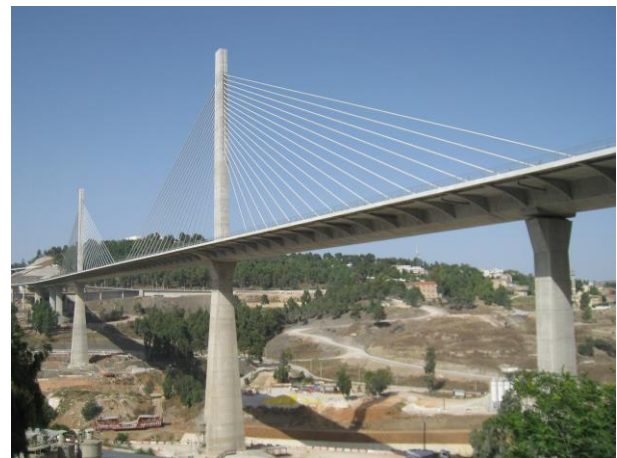
Figure 2. General view of the Salah Bey Viaduct
