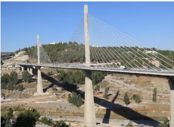
Figure 2. General view of the Salah Bey Viaduct
