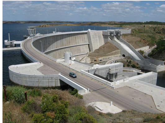
Fig. 1 Downstream face of Alqueva dam.
