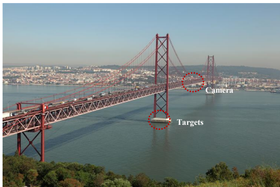
Figure 4. P25A suspension bridge in Lisbon (Portugal).
