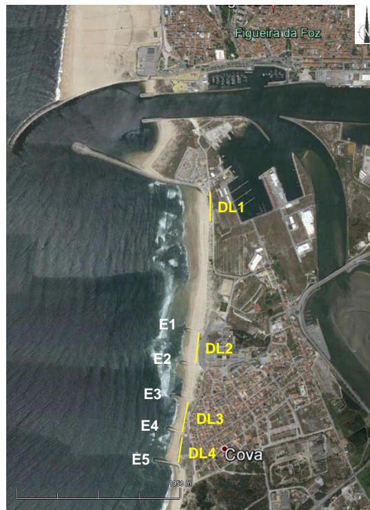
Figure 2.3 – Aerial photograph (18/6/2018; © Google Earth) of the Mondego river mouth and the coastal stretch of Cova-Gala, with its four alongshore defence structures (from DL1 to DL4) and five groynes (from E1 to E5)
