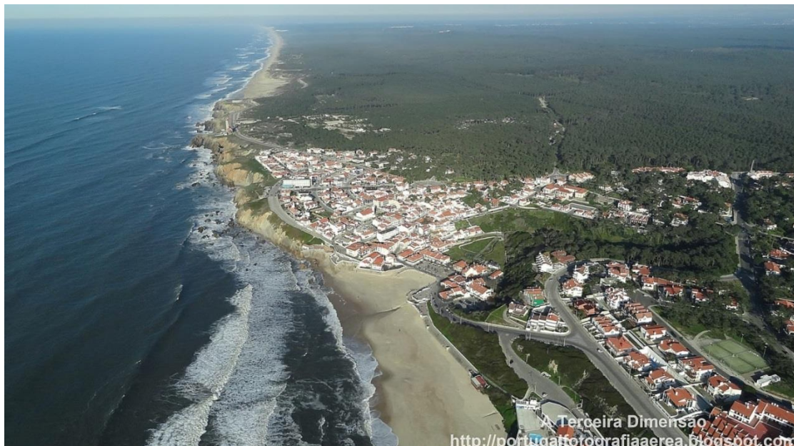
Figure 2.13 – Oblique aerial view of the seafront of São Pedro de Moel beach
