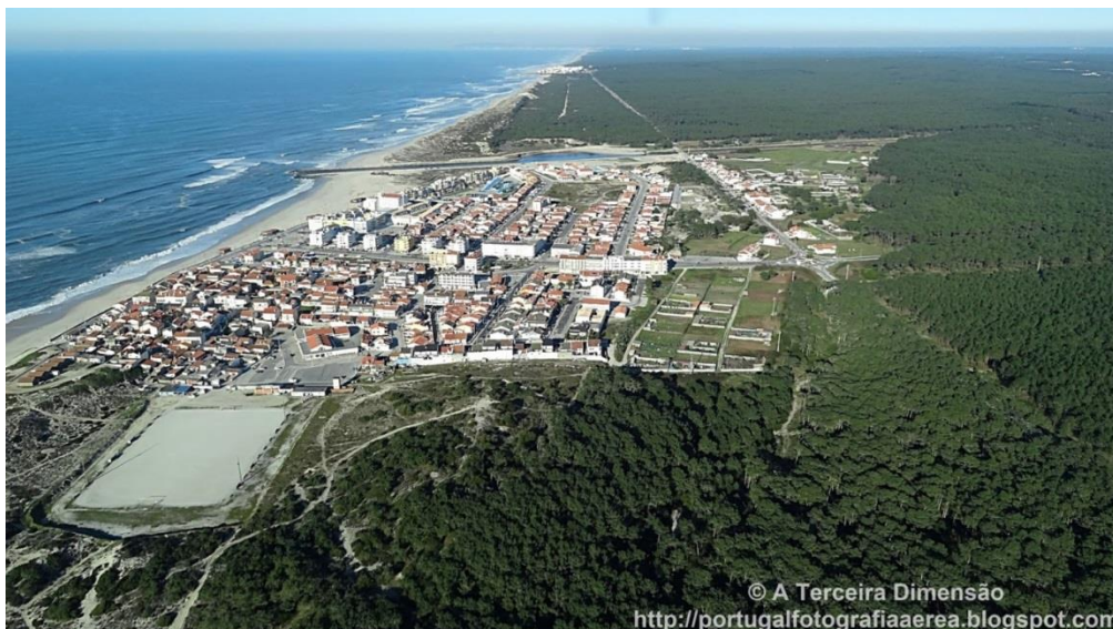
Figure 2.9 – Oblique aerial view of the seafront of Vieira beach
