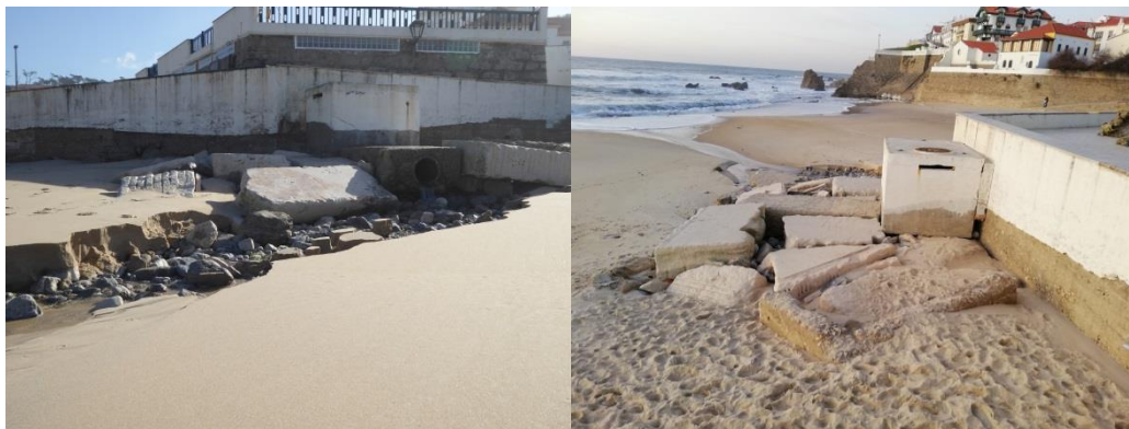
Figure 2.15 – Photographs of the São Pedro stream outlet and induced local erosion in São Pedro de Moel beach (Feb/2019)
