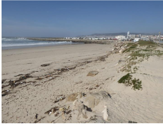
Figure 2.4 – Photographs of Cova-Gala beach: view of the south jetty of the Mondego river mouth from the dune at the northern extreme of the beach (25/Feb/2019)
