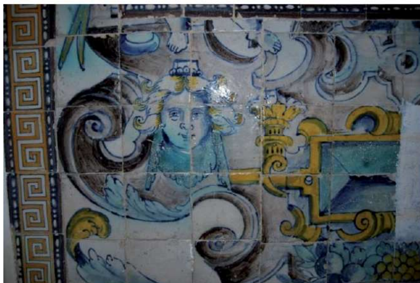
Figure 2: Part of an azulejo panel at Igreja da Graça in Lisbon. At the corners where the glaze detached, the underlying cream or reddish ceramic body became visible.
