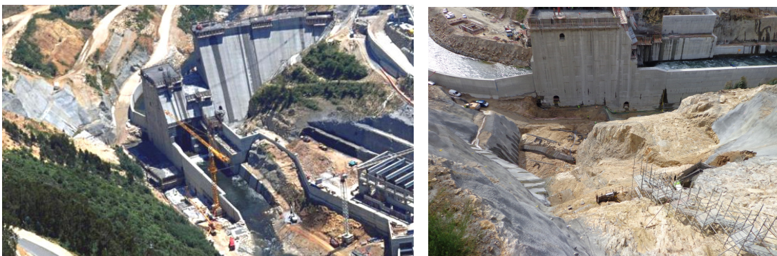
Figure 4: View of the site works and excavations on right bank in 2013
