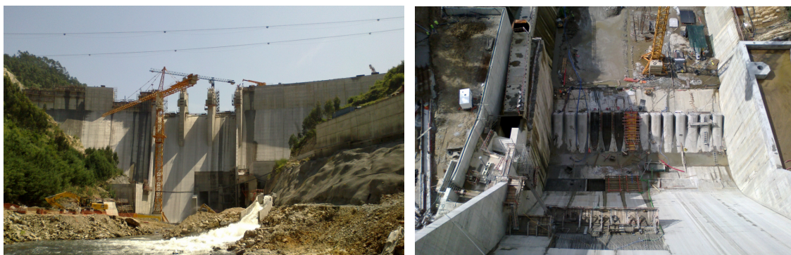
Figure 5: View of the dam site works and roller-bucket construction in 2014
